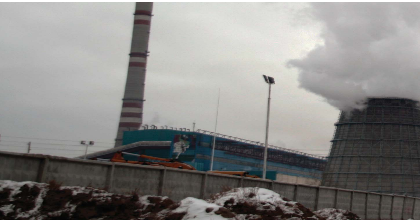
Combined heat and power station-4, 2011. Photo by Ts.Batbaatar
